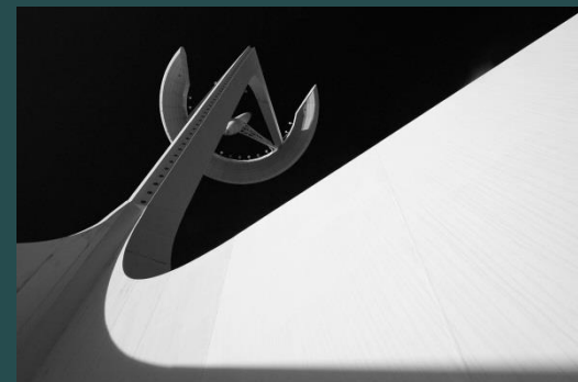
TELEFONICA TOWER WOLFRAM ERHARD WILDNER GERMANY
