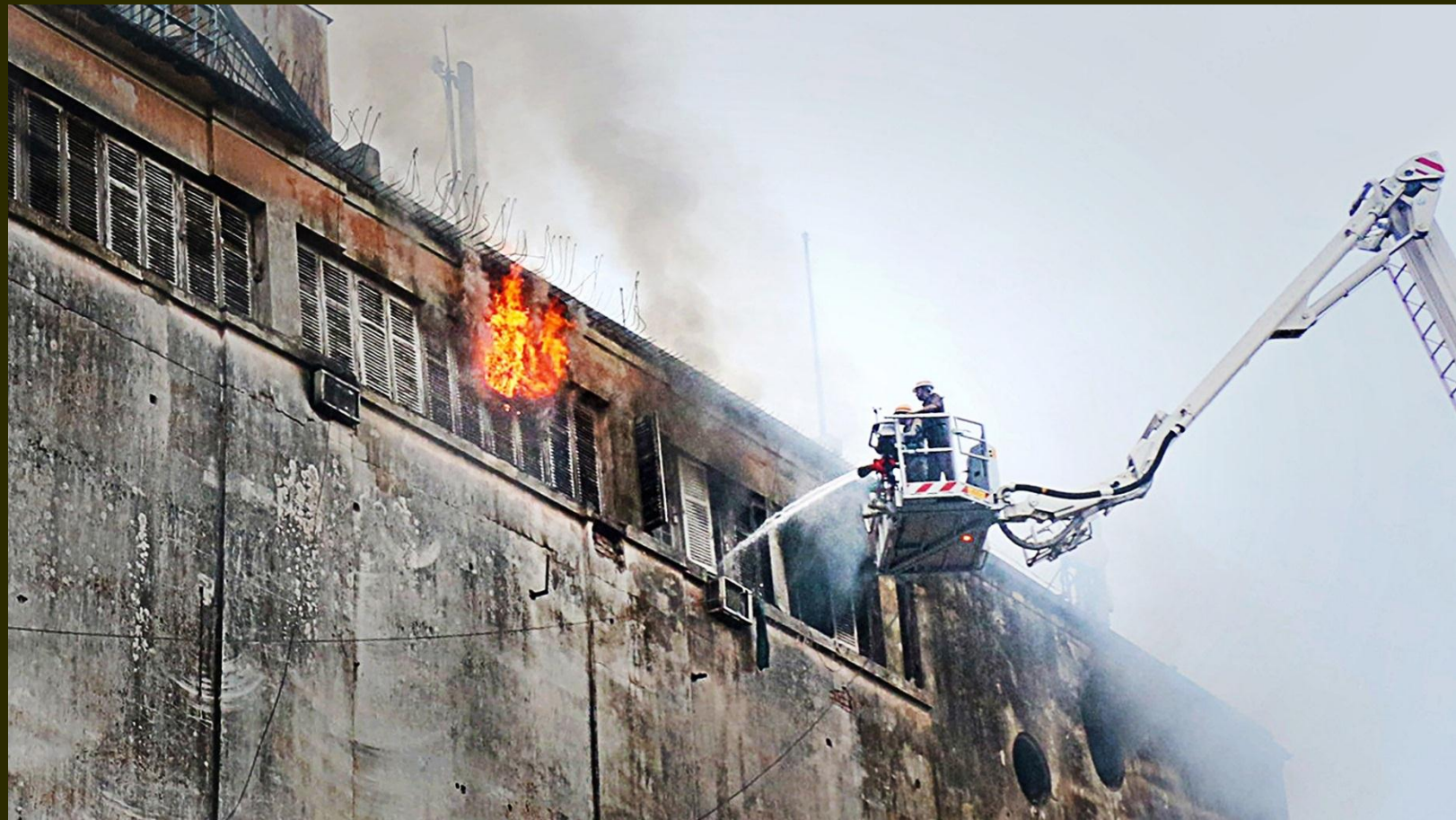
WATER SPRAY FOR FIRE
