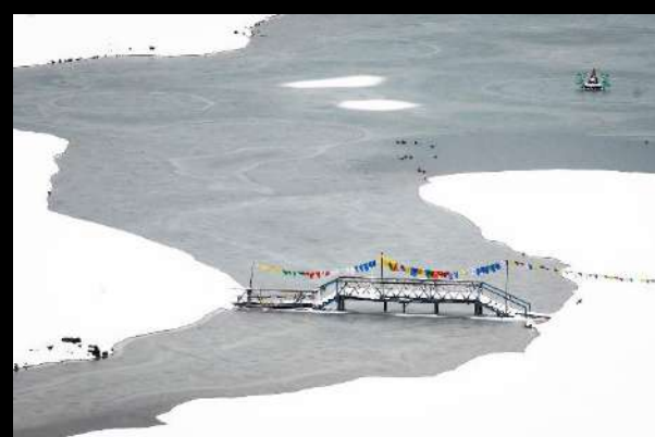
BRIDGE OVER FROZEN LAKE
