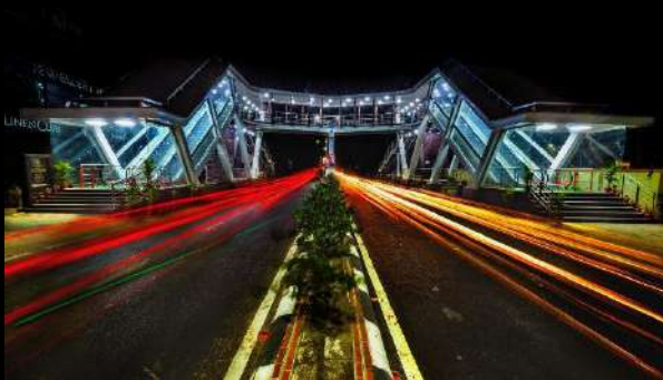
FOOT BRIDGE MANABENDRA BHATTACHARJEE
